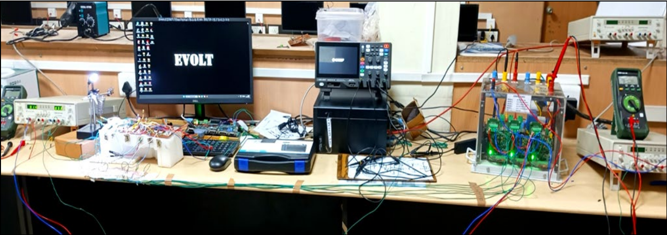
Fig 4: Complete experimental setup showing the three-phase induction motor, IGBT inverter, TMS320F28335 DSP controller, isolation and amplification circuits, and the 525V DC link power supply.
