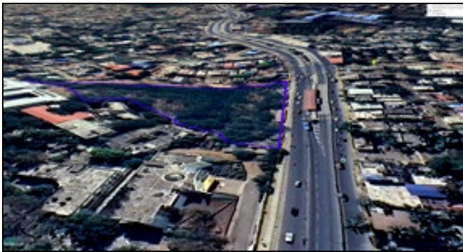
Fig 32: The existing condition of the road, footpath and pond
